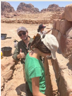
Lime mortar repair
